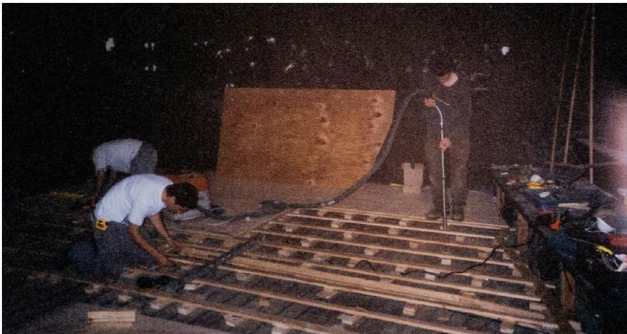
Figure 73: 2002. Stables Theatre Renovations. Source: SBW Foundation Archives.
